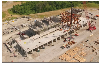
Construction of the Ark Encounter theme park, slated to open in July, is underway in Kentucky. (photo courtesy of Answers in Genesis)
